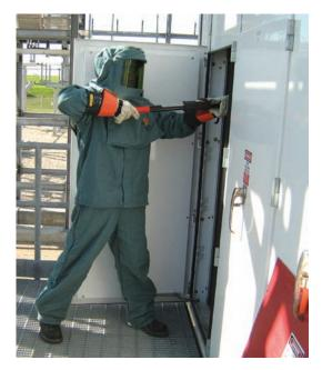
**Figure 1-4** An arc flash hazard exists when a person interacts with equipment. © Chemco Electrical Contractors Ltd.
